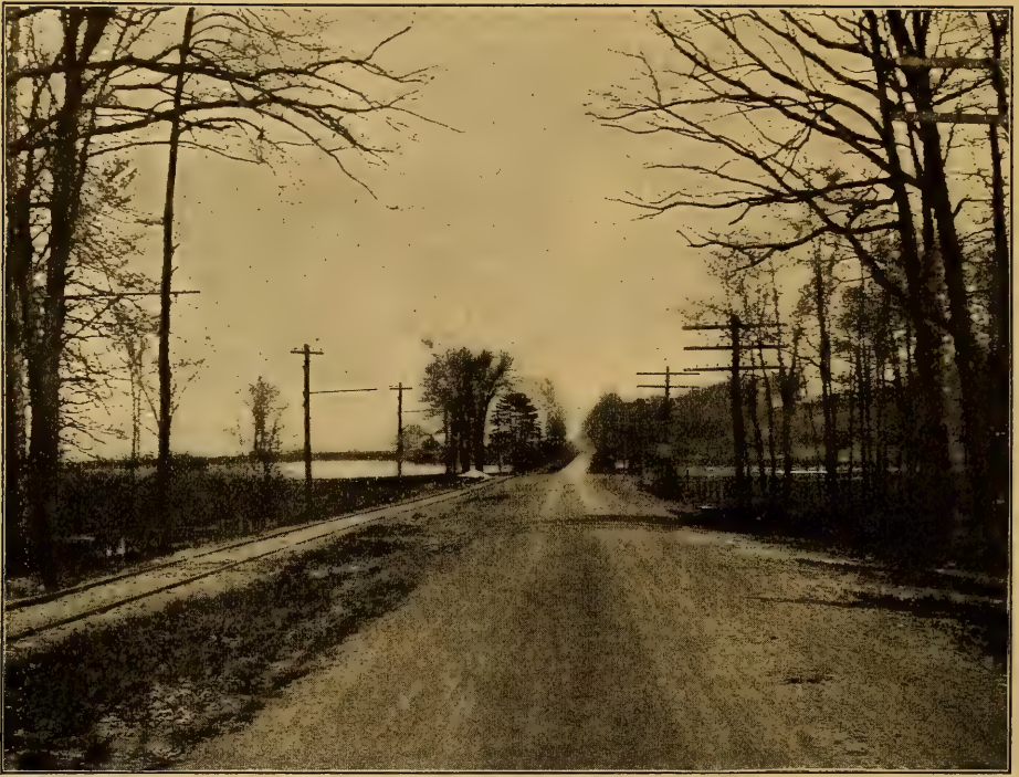
Farmington Road, in Connecticut, treated with a coal tar preparation to prevent formation of dust.
